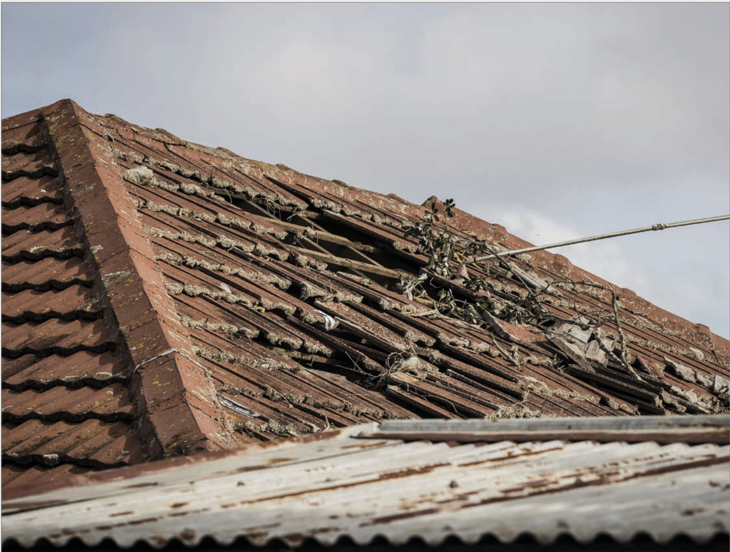
Roof damaged by Auckland tornado. Photo: RICKY WILSON/STUFF
